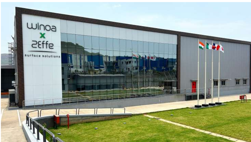
Front view of the new shot-peening center
